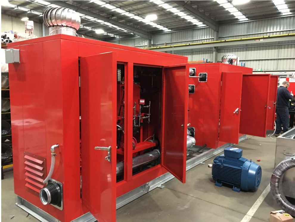
Double diesel enclosure inline on base
