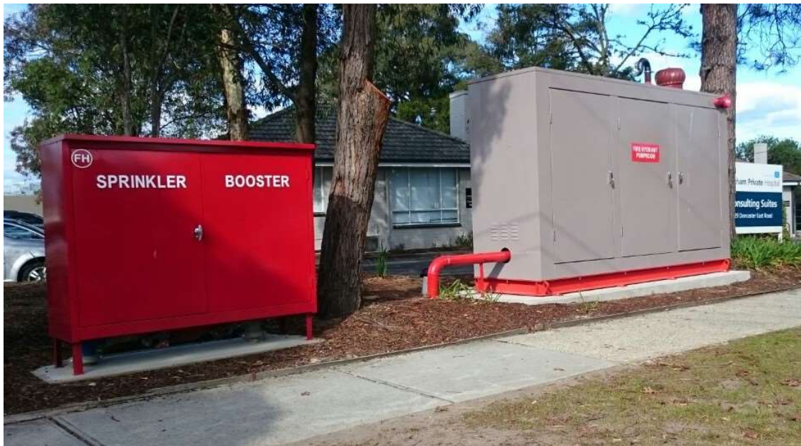
Single diesel enclosure unit on site
