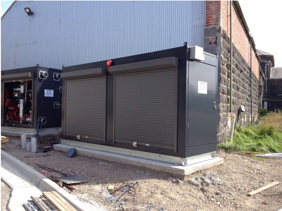
Single diesel enclosure unit with roller doors
