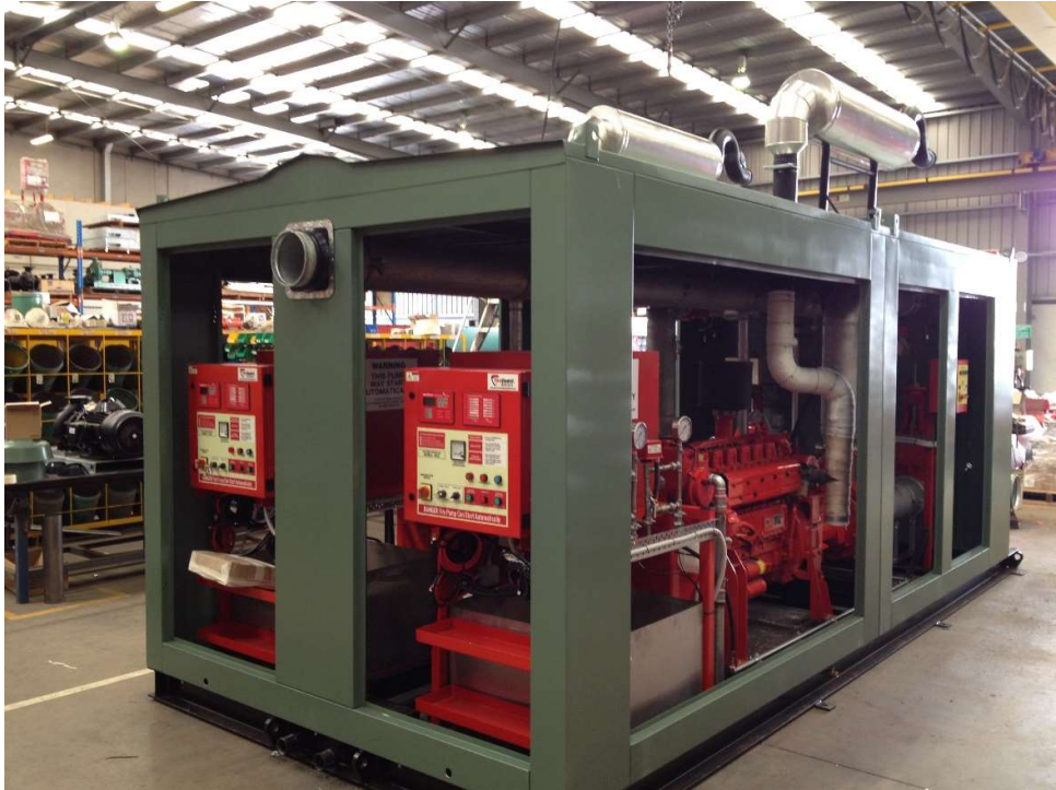
Double diesel enclosure unit (doors not installed)
