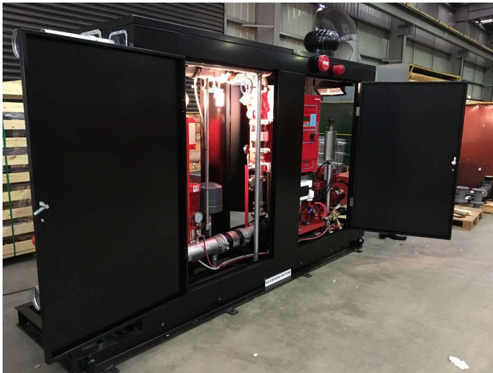
Single diesel enclosure unit
